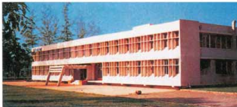
Manufacturing and Research & Development Centre, Navi Mumbai
